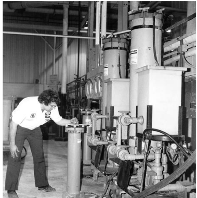
Filter cartridges are changed only when pressure (being checked by Mike Griebel) exceeds 40 psi. Normally this occurs only twice a year.
