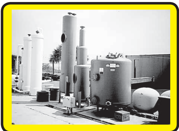
SALTWATER FISH FARM - BACTERIA TOWER, AERATION TOWER & FILTER SYSTEM
