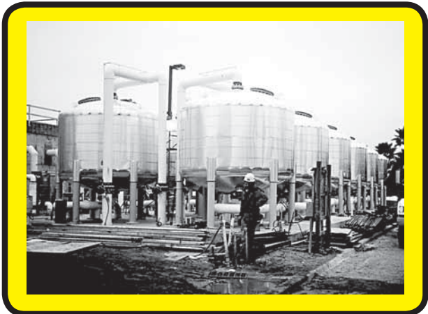
SALTWATER FISH FARM - BACTERIA TOWER, AERATION TOWER & FILTER SYSTEM
